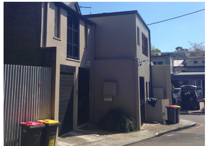
Figure 3 - View of properties with frontages to McPherson Lane
